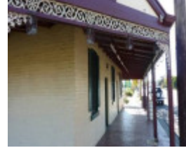
Detail of external wall at corner of High and View streets.
