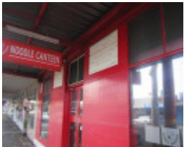
Detail of the west elevation.
