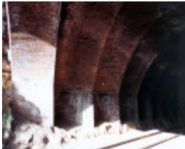
B7683 Dandenong Road Railway Bridge Underside 3
