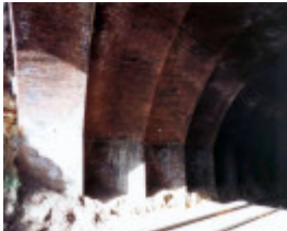
B7683 Dandenong Road Railway Bridge Underside 3
