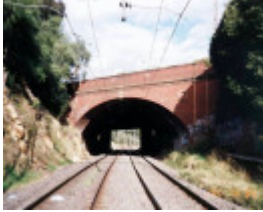
B7683 Dandenong Road Railway Bridge
