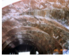
B7683 Dandenong Road Railway Bridge Underside 2
