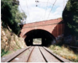
B7683 Dandenong Road Railway Bridge
