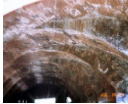
B7683 Dandenong Road Railway Bridge Underside 2
