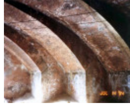
B7683 Dandenong Road Railway Bridge Underside 1
