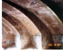
B7683 Dandenong Road Railway Bridge Underside 1
