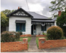
4 Kilmuir Road, Malvern East
