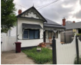
6 Kilmuir Road, Malvern East
