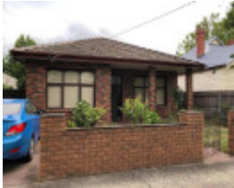
10 Kilmuir Road, Malvern East
