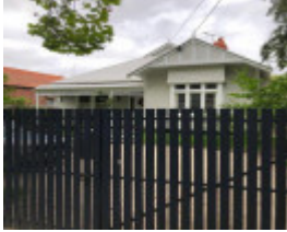
29 Warley Road, Malvern East
