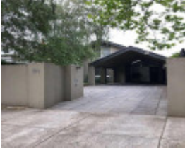
31 Warley Road, Malvern East
