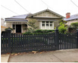
37 Warley Road, Malvern East
