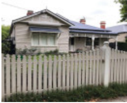
39 Warley Road, Malvern East
