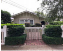
6 Warley Road, Malvern East
