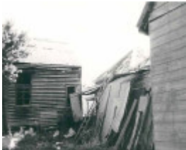
B3226 Parslow's House Rear View
