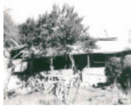
B3226 Parslow's House Front View
