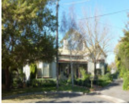
West elevation of Myrnong.
