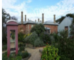
West elevation, viewed from Morrison Street.
