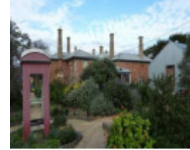
West elevation, viewed from Morrison Street.
