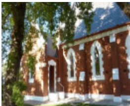
Entry to the sacristy (north elevation).
