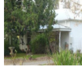
Detail of verandah.
