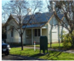
South east elevation of the front to Camp Street.
