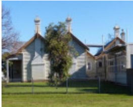
East elevation of the police station and quarters, showing the three 1880s transverse gables.
