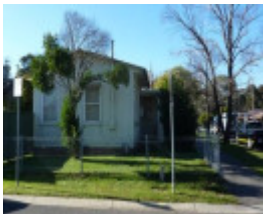
West elevation of the freestanding 1963 addition at the south-west corner of the site.
