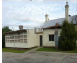
Rear view of the police station and quarters, with the classroom addition at left (east).
