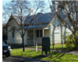
South east elevation of the police station and quarters, showing the front to Camp Street.
