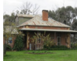
South-east elevation, note timber dormer at rear.
