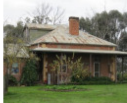
South-east elevation, note timber dormer at rear.
