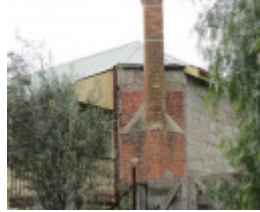
Brick chimney at chamfered corner, possibly a former entrance.
