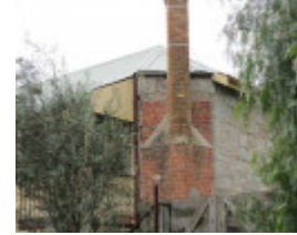
Brick chimney at chamfered corner, possibly a former entrance.
