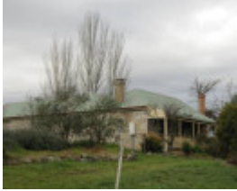
North elevation, as seen from the Calder Alternative Highway.
