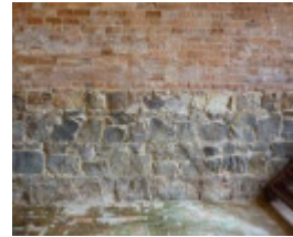
Footings of outbuilding, possibly 1860s.
