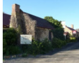
The 1860s wing; note stepped chimney form.
