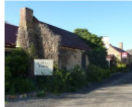
The 1860s wing; note stepped chimney form.
