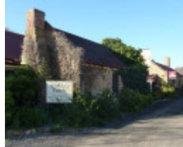
The 1860s wing; note stepped chimney form.
