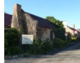
The 1860s wing; note stepped chimney form.
