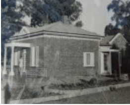
Byronsvale (then Turand), c. 1950s, following renovations (Source: Private collection, Pat and David Andrew).
