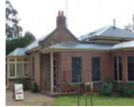
Byronsvale looking west, note new entrance porch to 1872 wing (left), and additions to the west elevation.
