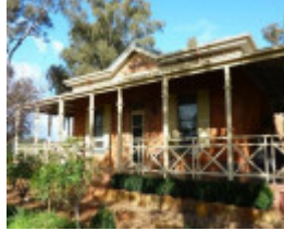
North elevation, note recent verandah.
