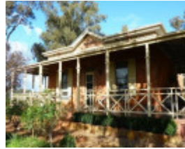
North elevation, note recent verandah.
