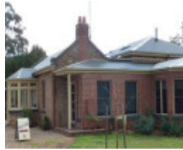
Byronsvale looking west, note new entrance porch to 1872 wing (left), and additions to the west elevation.
