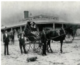
The original Shamrock Hotel, undated, viewed from the north-east.
