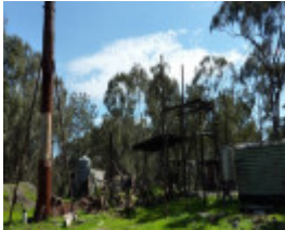
From left, looking north: Metal stack; remnants of brick boiler housing; gantry for truck-mounted vat; and rail carriage (former eucalyptus cutter's hut).
