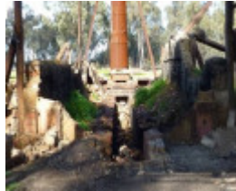
Brick housing for boiler, removed 2010.
