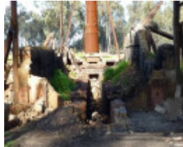
Brick housing for boiler, removed 2010.
