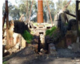
Brick housing for boiler, removed 2010.
