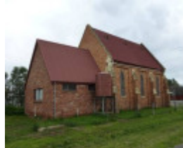
Addition at the rear of the church.
