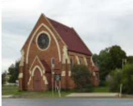
West and north elevations. Note bell tower to the north (right) of the church.
