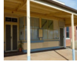
Shopfronts, note two doors and signage ('Confectionary' and 'Soft Drinks') to upper windows.
