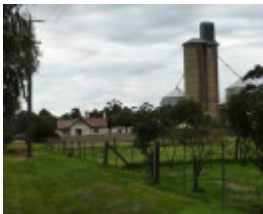
East elevation, with grain silo at rear.
