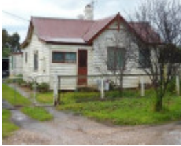
South elevation. Note infilled verandah to the west of the projecting gable.
