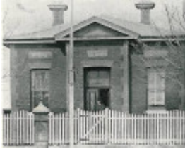
Raywood Town Hall north elevation, c. late-19th century
