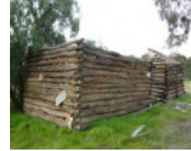
View of site from Rothackers Road (west)
