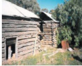
View of the two stores from the north
