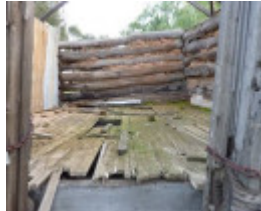
Raised floor and remnant mud and brick pugging to the eastern store
