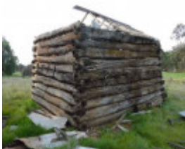
The eastern store, viewed from the south-west
