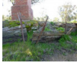
Section of the timber retaining wall.
