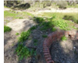
Brick vats adjacent to the stack.
