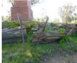
Section of the timber retaining wall.
