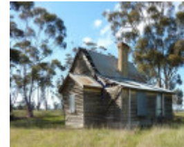
North and west elevations, note sugar gums at rear.
