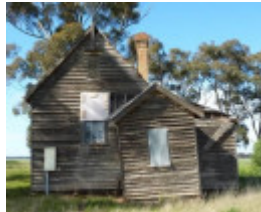
North elevation of the Former Kamarooka Road School.
