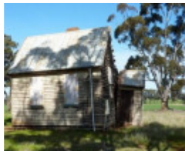
West elevation, note partially detached entrance porch.
