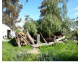
The entry to the former larder (east face).
