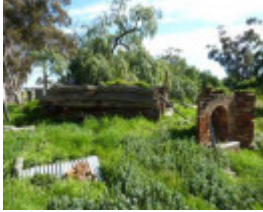
South side of the former store, with the fireplace of the former house at right.
