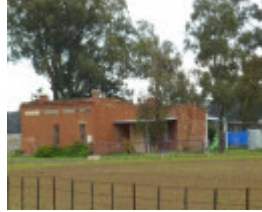
Former Royal Hotel, rear (east)
