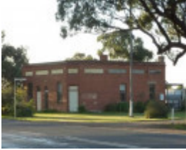
Former Royal Hotel, south and west elevations viewed from the Loddon Valley Highway
