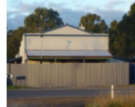
Former Old House at Home Hotel, west elevation, note tall corrugated sheet metal boundary fence
