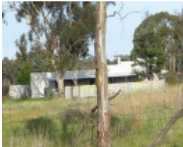
Former Old House at Home Hotel, north elevation, viewed from Camp Road
