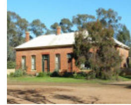
Former Camp Hotel and Store, east elevation
