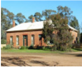
Former Camp Hotel and Store, east elevation
