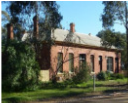
Former Camp Hotel and Store, east elevation
