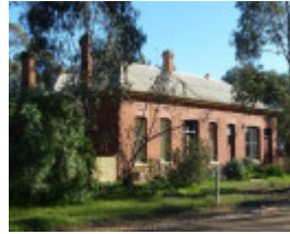
Former Camp Hotel and Store, east elevation
