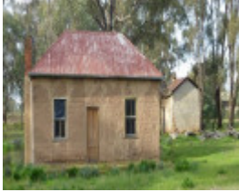
Kelly Cottage, front (west) elevation, with gable roofed outbuilding at right (south)
