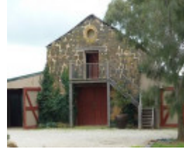
Barn/store to the north of the house.
