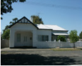
Former Post Office and Residence
