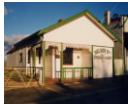
Historical Society Resource Centre after restoration, n.d. Source: Linton Historical Society
