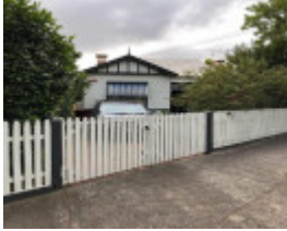
14 Warley Road, Malvern East
