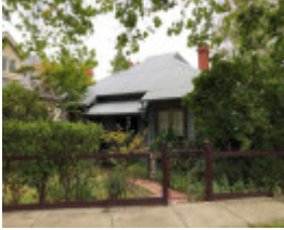
18 Warley Road, Malvern East
