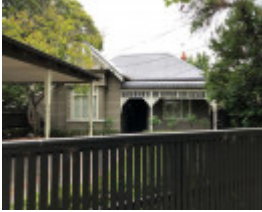
22 Warley Road, Malvern East
