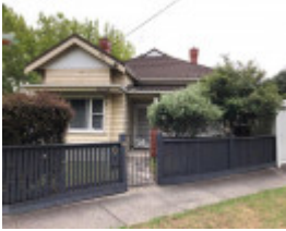
24 Warley Road, Malvern East
