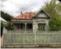
10 Moama Road, Malvern East
