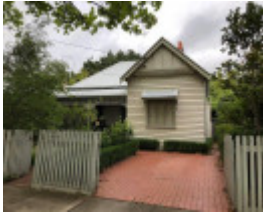
12 Moama Road, Malvern East
