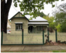
14 Moama Road, Malvern East
