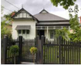
20 Moama Road, Malvern East
