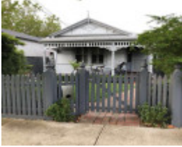
34 Moama Road, Malvern East
