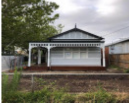
36 Moama Road, Malvern East
