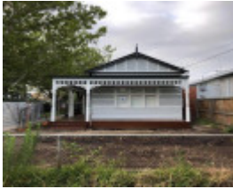
36 Moama Road, Malvern East
