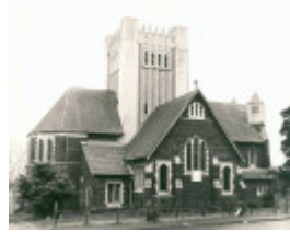
B3402 St Andrew's Church NE View
